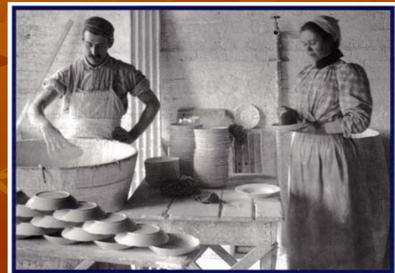
Onondaga Pottery workers dipping ceramic ware into vats of glaze, ca. 1899.
