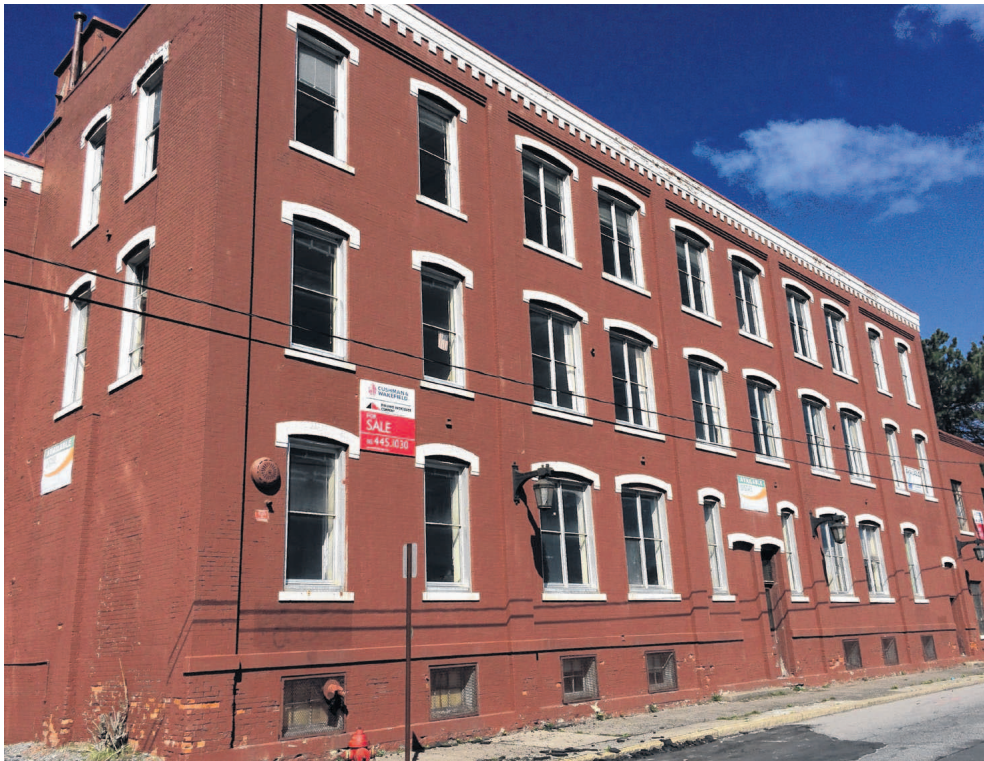
Developer Norm Swanson plans to turn the former Syracuse Lighting Co. headquarters, at 311 Genant Drive in Syracuse's Franklin Square neighborhood, into a beer garden restaurant, a microbrewery and a tasting room for New York beers, wines and foods. (Rick Moriarty / r Moriarty@syracuse.com)
