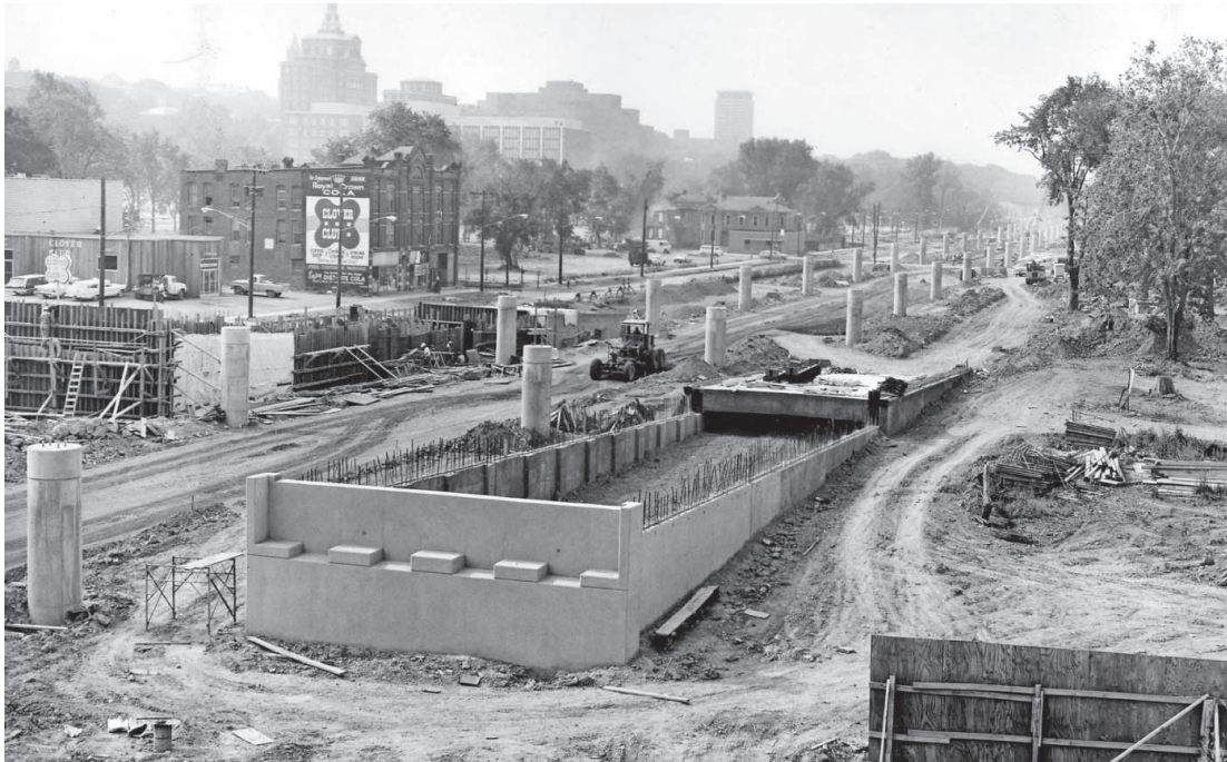
Construction of Interstate 81 along Almond Street, looking south from downtown Syracuse, in the 1960s. Crouse Hospital's clock tower is in the distance. Clover Club, a jazz club, is one-story building at left. Onondaga Historical Association
