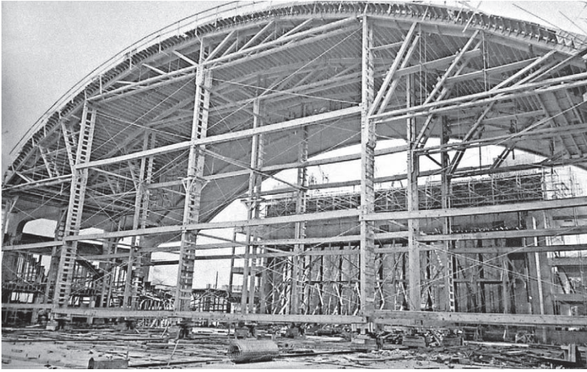
The Onondaga County War Memorial under construction in June 1950.
