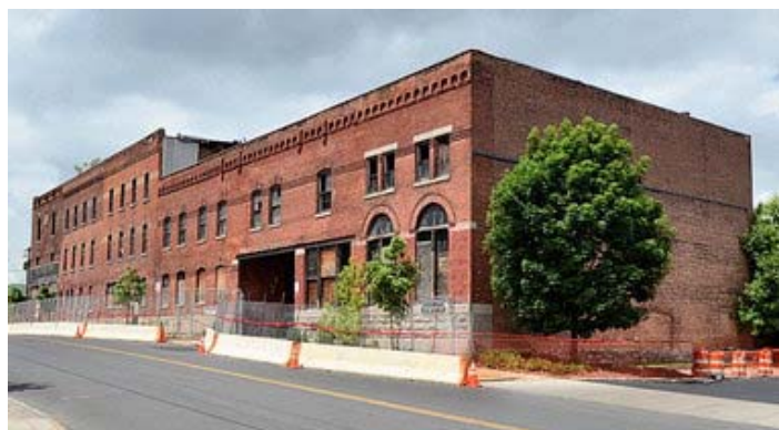
The historic Otisca Building, site of a brewery for many decades, shortly before its demolition in May. Housing Visions plans to build Otisca Commons, a three-story building with commercial space and 20 apartments, on the site.
