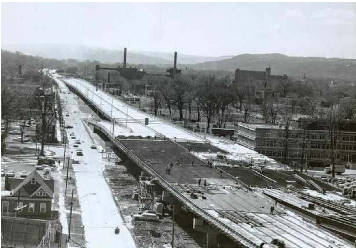
Construction of Interstate 81 through Syracuse, circa 1965. (Courtesy of the Onondaga Historical Association)
