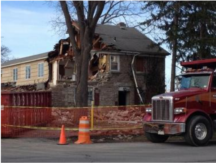
Demolition this week of the old Geddes farm
