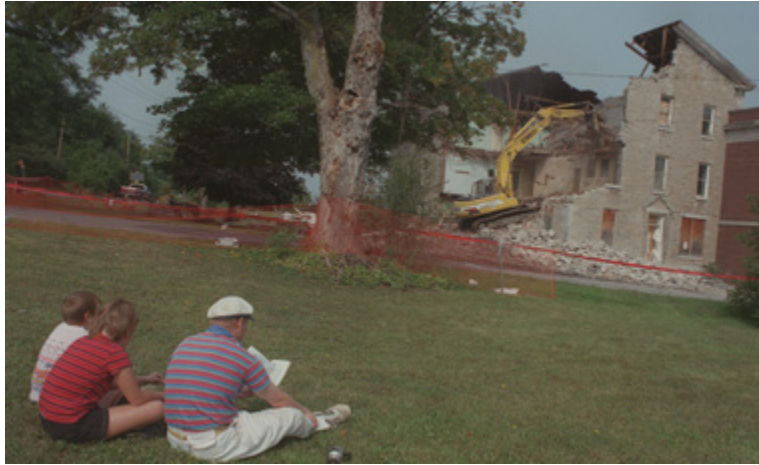
The demolition of the old Onondaga County poorhouse, in 1998:
