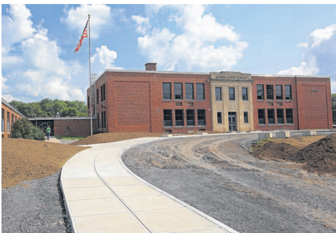
The council is seeking a $200,000 grant to help the Woodbine Group build the $2 million Tailwater Barn, a 10,000-square-foot, full-service banquet facility at Tailwater Lodge in Altmar. The lodge was converted from a former school. (Dick Blume / ddblume@syracuse.com, file)
