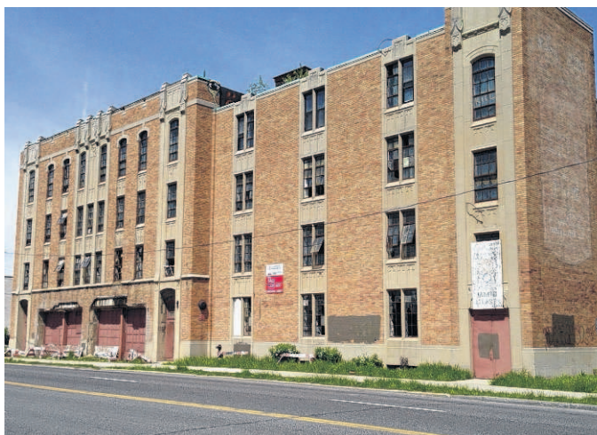
A development group plans to turn the C.G. Meaker Food Co. Building at 538 Erie Blvd. W. In Syracuse into 33 apartments and commercial space. The council is seeking a $1 million state grant for the nearly $6 million project, which will continue the revitalization of the Park Avenue neighborhood. (Rick Moriarty / rmoriarty@syracuse.com, file)
