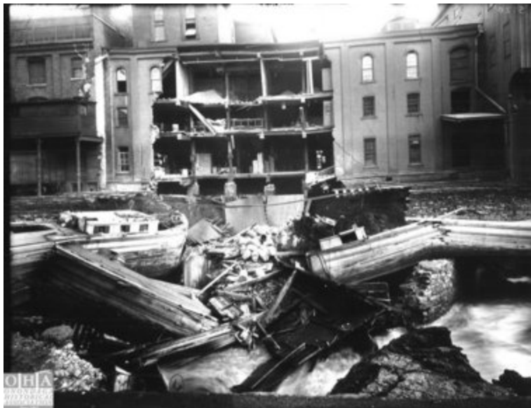
The great collapse of 1907: A mill wall fell into the
