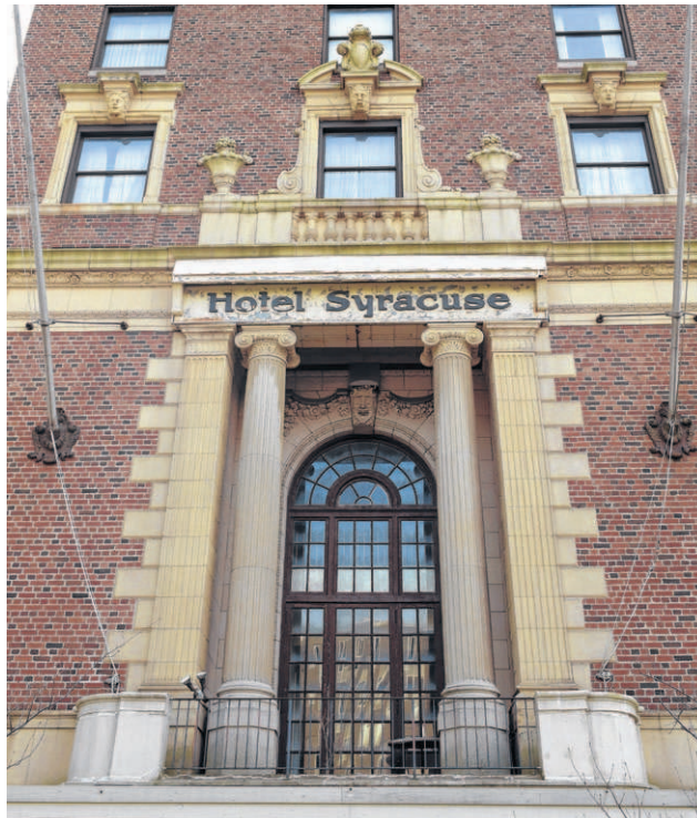
The Hotel Syracuse, which opened in 1924, is undergoing a restoration. (David Lassman / dlassman@syracuse.com )
