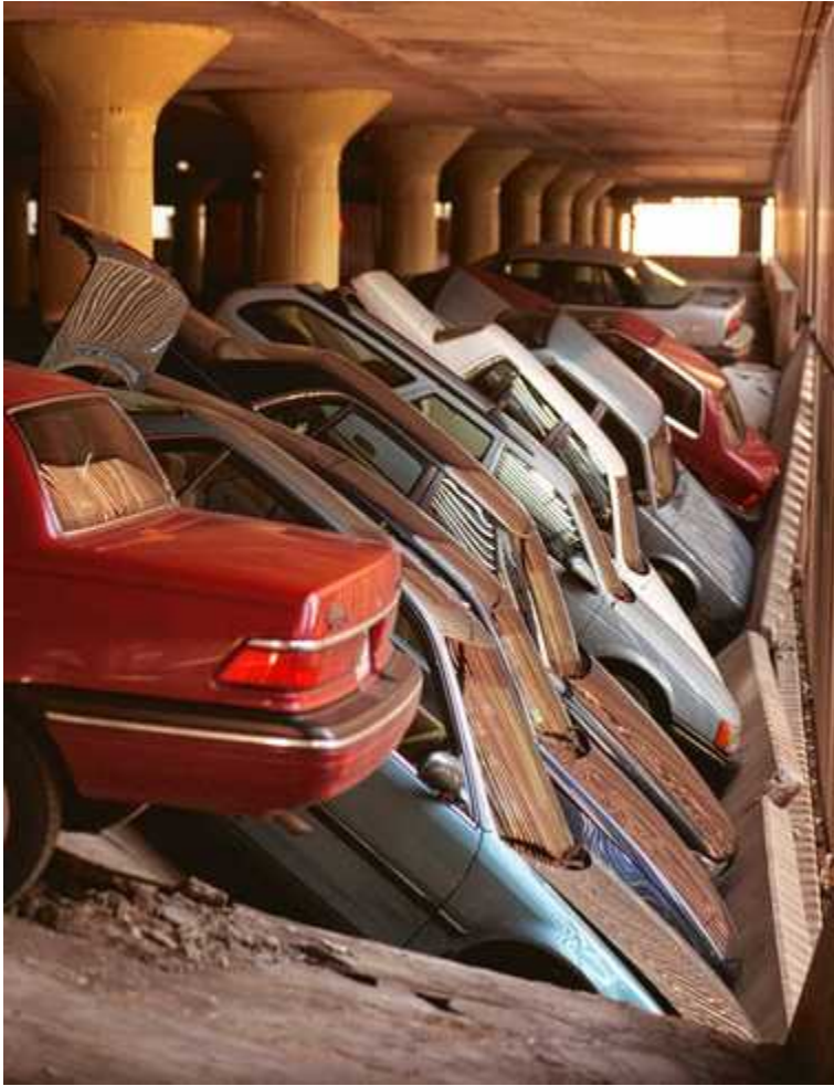
Here's what the MONY parking garage looked like when the second floor collapsed. Eventually, most of it was torn down to make way for The Tech Garden. 1994 file photo / Tom Fedor
