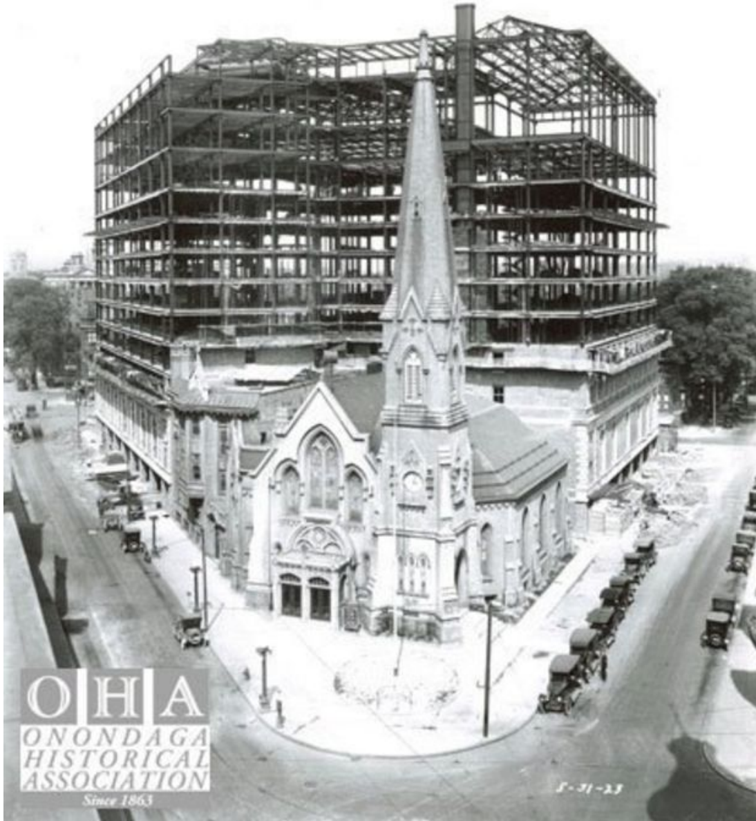
The Hotel Syracuse, under construction in the 1920s at the corner of Harrison, East Onondaga and South Salina streets. In the foreground is the Fourth Presbyterian Church, built in 1877. The church was torn down to make way for a parking lot in 1943. Onondaga Historical Association | Submitted image
