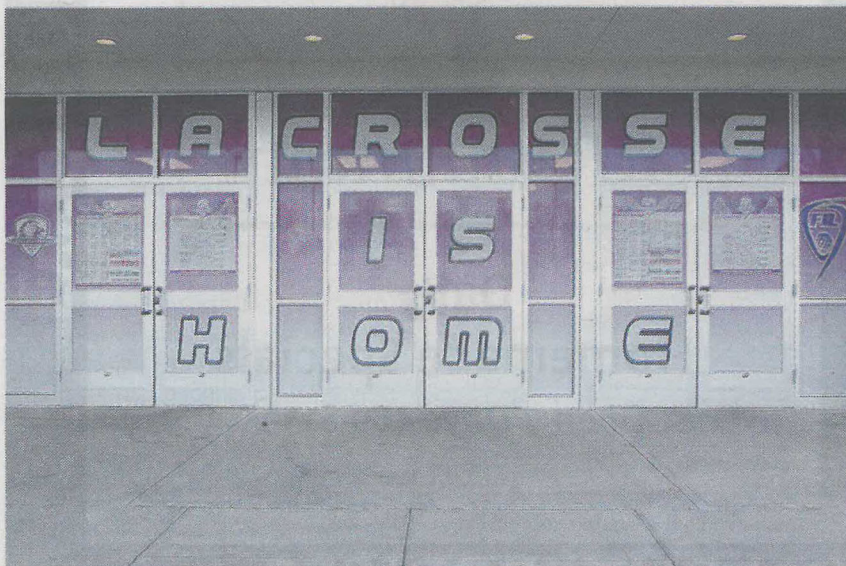
The entrance to the Tsha'hon'nonyen'dakhaw' Ice/Lacrosse Arena.
