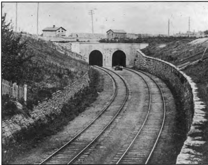
This old photograph depicts the original New York Central mainline underpass beneath the Erie Canal in Syracuse. It would have been there at the time of the Lincoln funeral train. After the canal was abandoned in 1917 to become Erie Boulevard East, it was replaced by a single-portal underpass.
