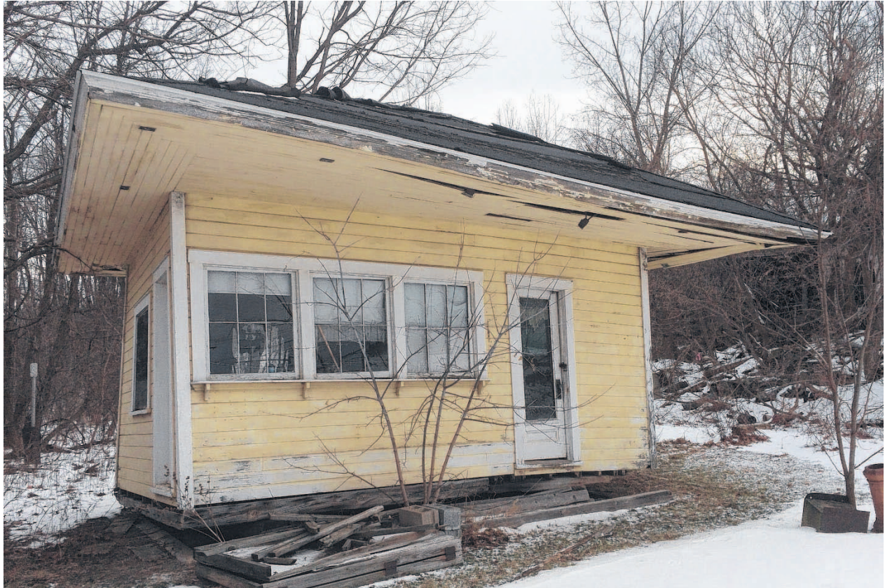
This building at 1001 E. Brighton Ave. in Syracuse looks like it might have been part of a railroad depot at one time. Developer Joe Hucko said he may preserve the building when he redevelops the property with a complex of office, retail and apartment buildings. (Rick Moriarty / rmoriarty@syracuse.com )
