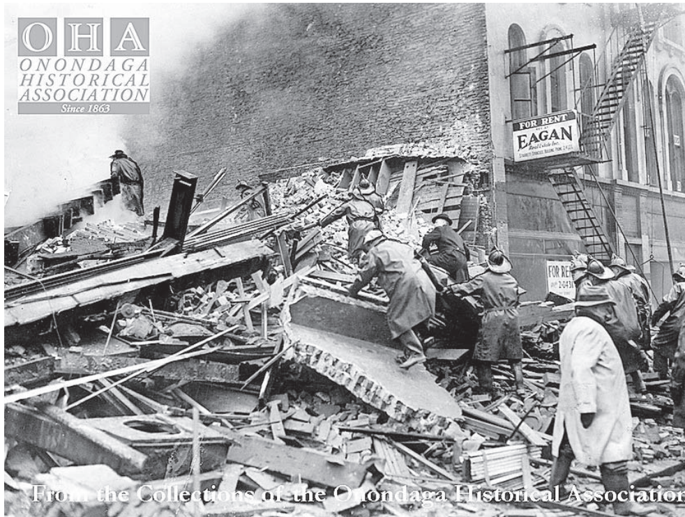
Firefighters begin to search the rubble of the Collins Block in an attempt to locate survivors after the building collapsed. Nine firefighters lost their lives when a floor gave way. Onondaga Historical Association photo
